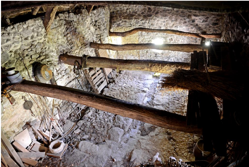
Figure 2: Higher Uppacott shippon drain from loft level
