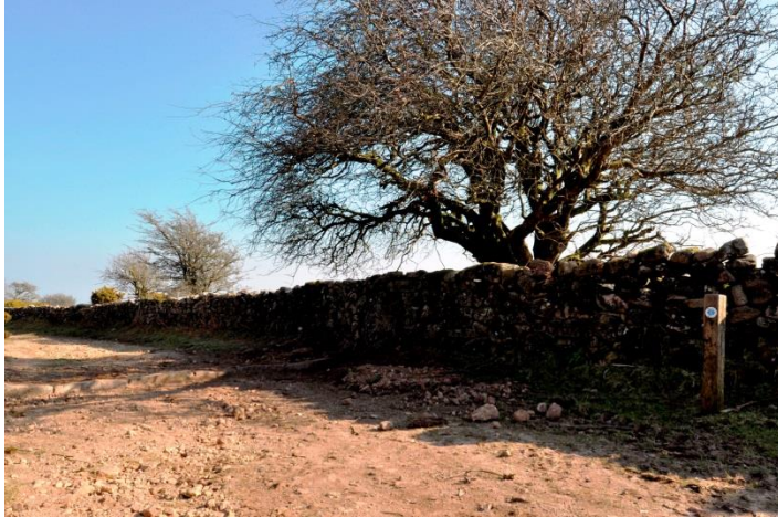
Bel Tor Driftway after repair work has been completed
