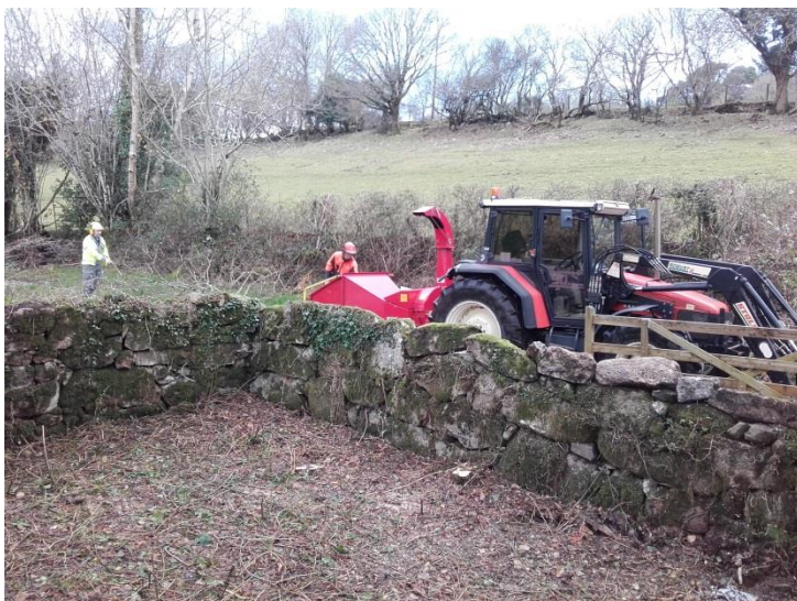
Poundsgate Pound repair work in progress
