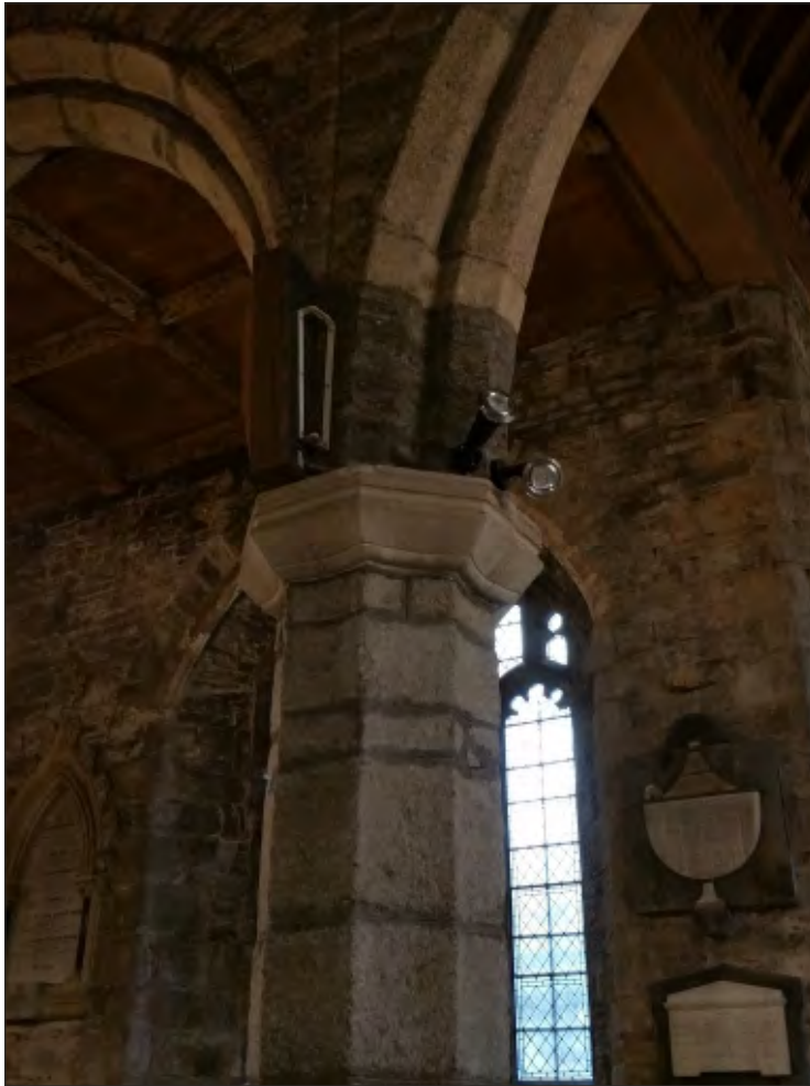
Fig. 10 Close-up of north crossing pier showing volcanic material at base of arch rather than granite highlighting the possible position of early 15th century rood screen. Looking northwest.
