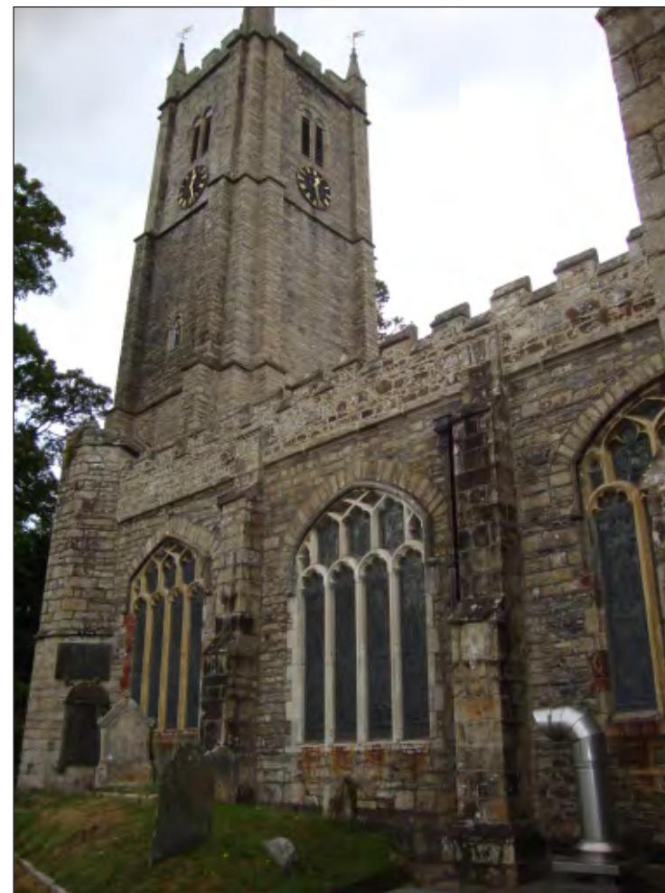
Fig. 5 General view of south aisle wall showing blocked doorway and later enlarged window. Looking northwest.
